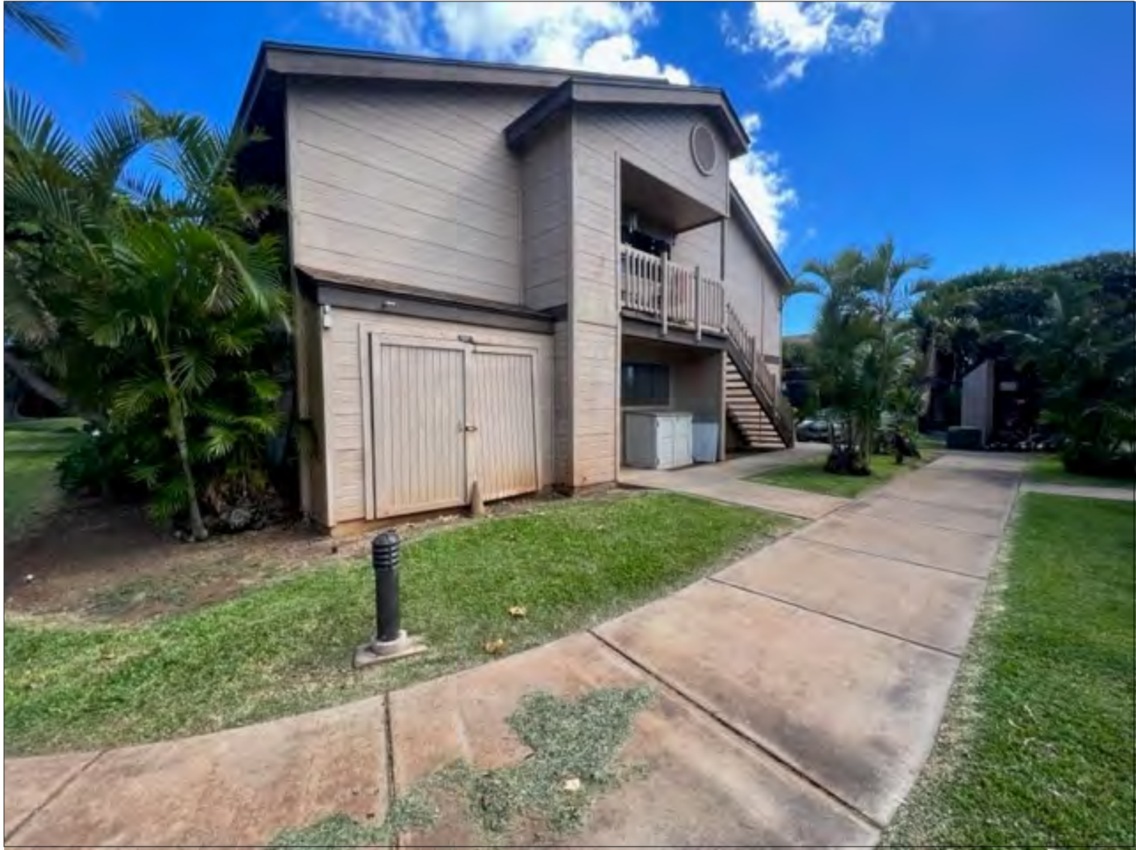
Building, Siding, Electrical Enclosure, Stairs, Railing, Walkway and Light Bollard
