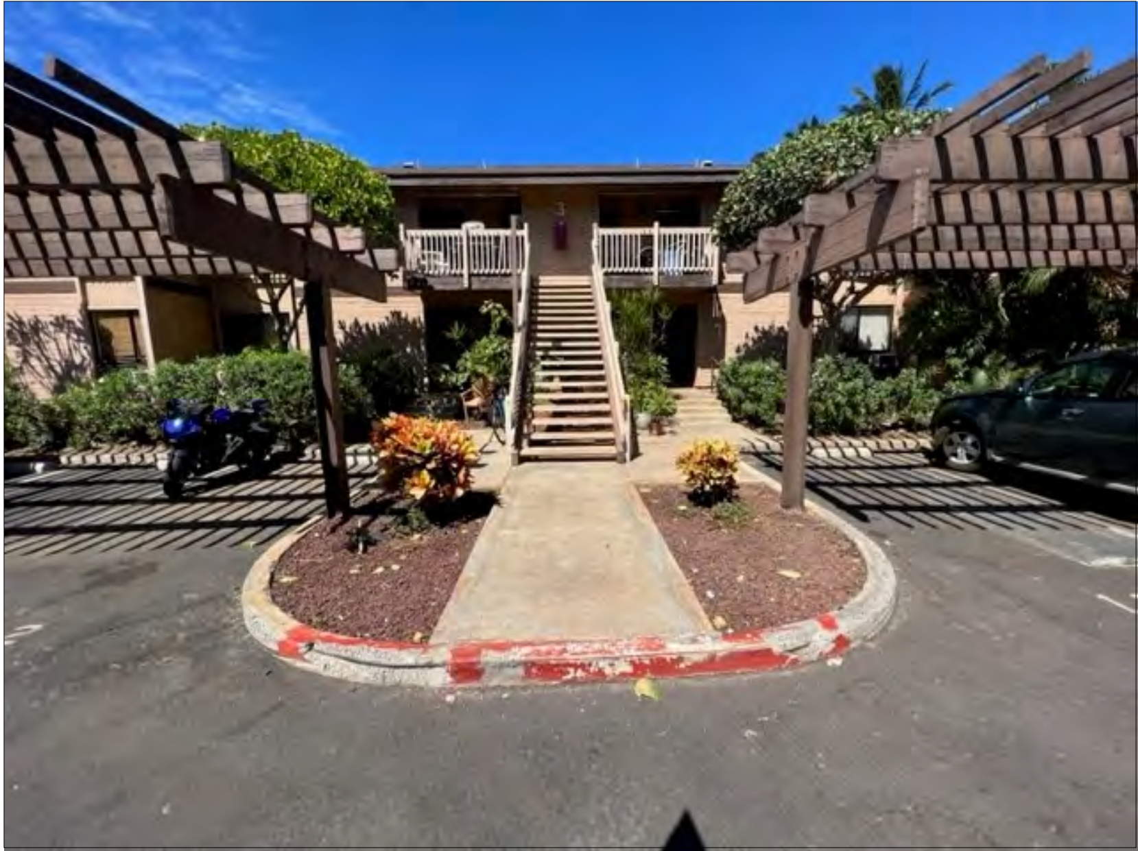
Second story stairs, railings, carport and curbing
