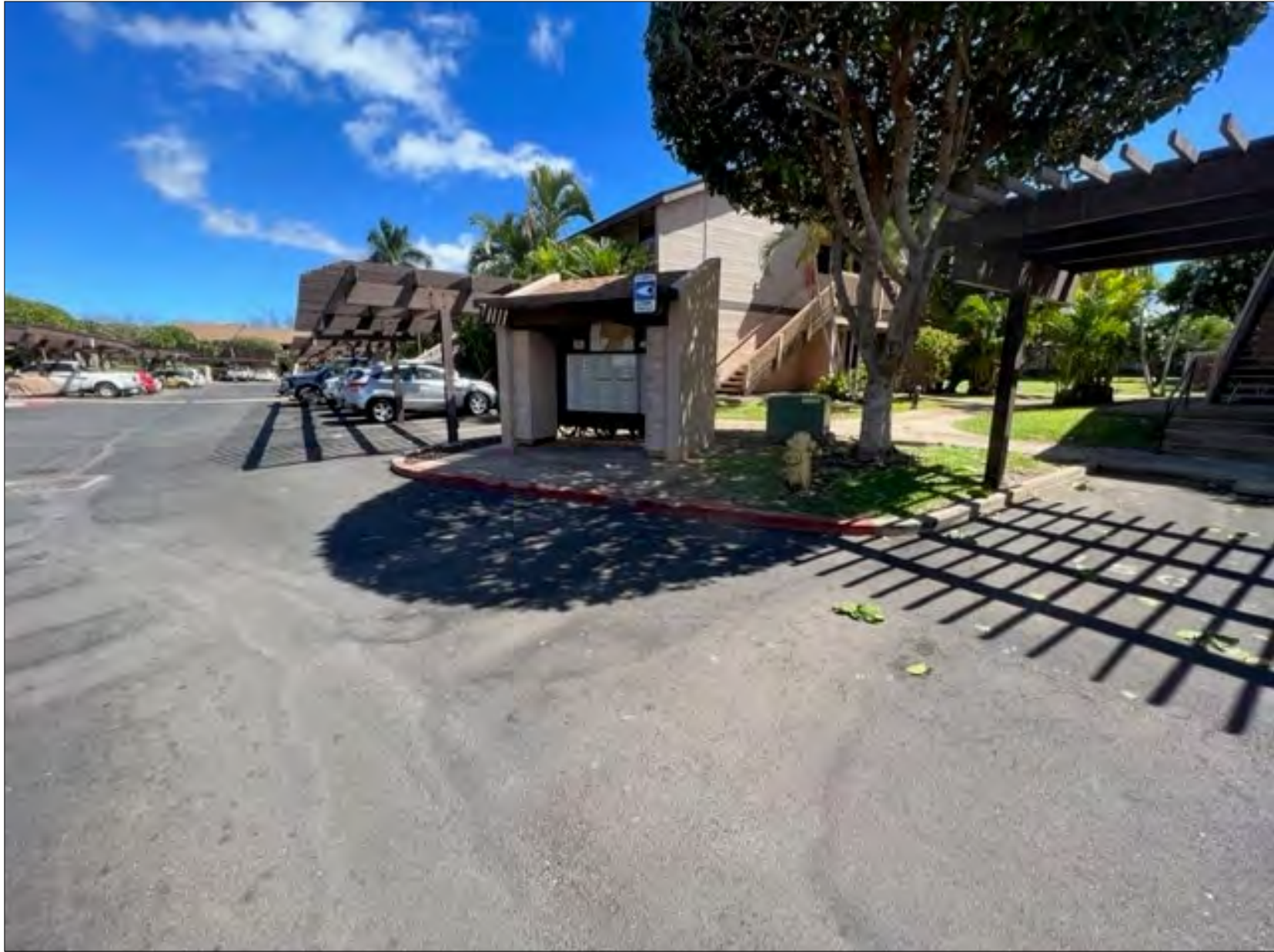
Mailboxes, Enclosure, Hydrant and Roadway
